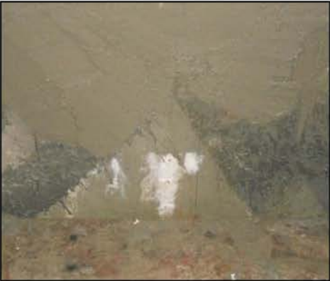
(b) 涌水灌浆堵漏后
