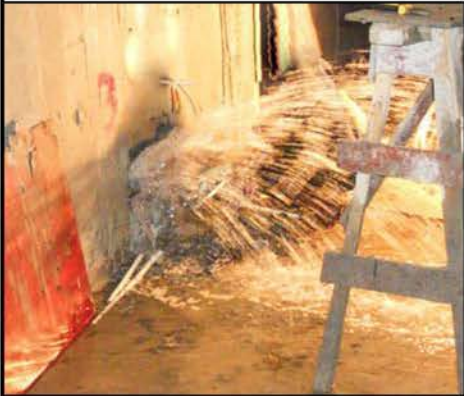
(a) 涌水灌浆堵漏前
